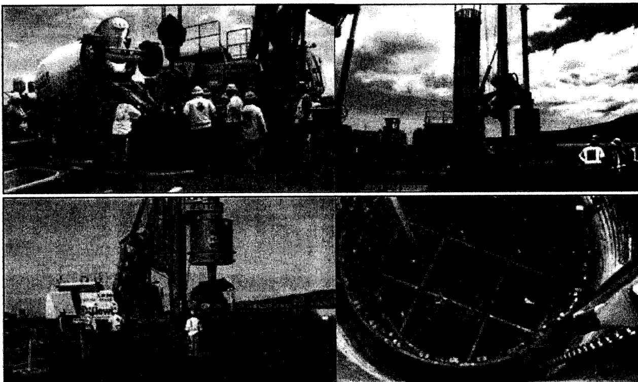
Figure 1. Pier 65 Foundation Shaft Placement
